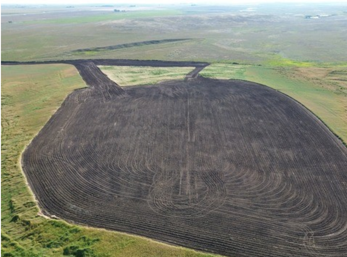
Grading Crews Completing Borrow Reclamation SE of RR 143 Looking East
