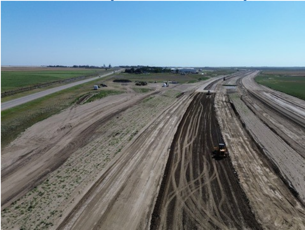
Grading Crews Completing Subgrade Prep in Bypass at RR 135 Looking East
