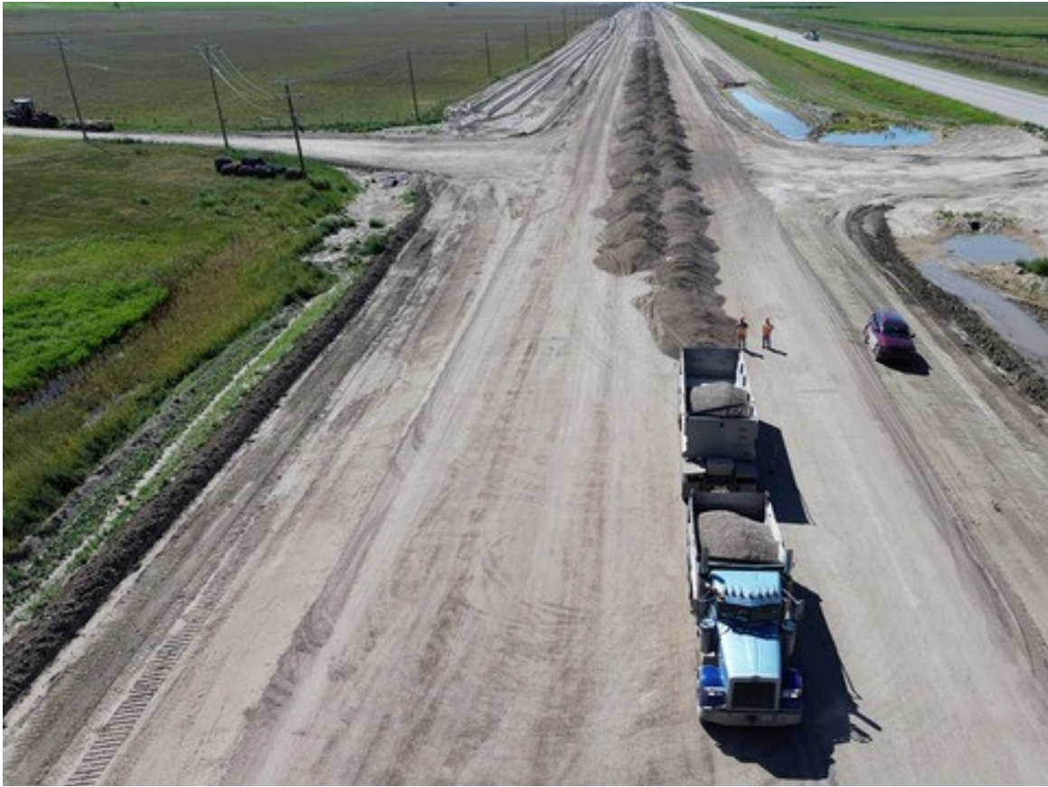
Base Crews Windrowing 2nd Lift of Gravel at RR 141 Looking West
