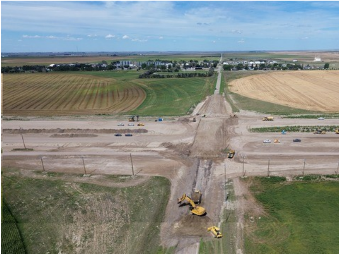
Grading Crews Completing HWY 877 Intersection Lowering South of Grassy Lake Looking North
