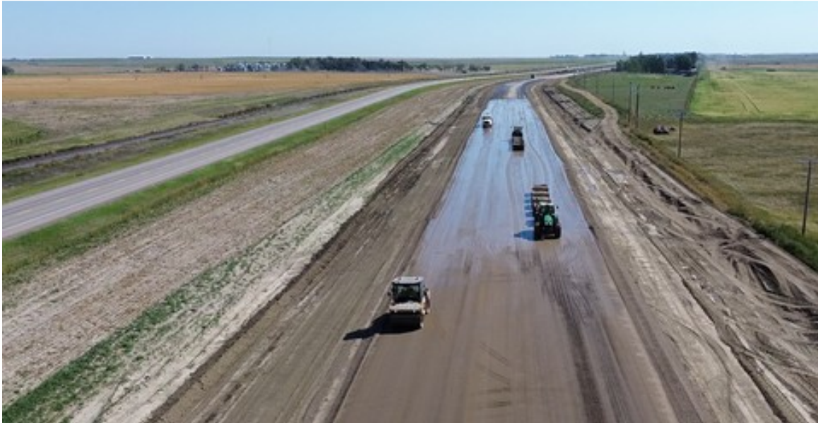
Base Crews Packing 2nd Lift of Gravel at RR 144 Looking East
