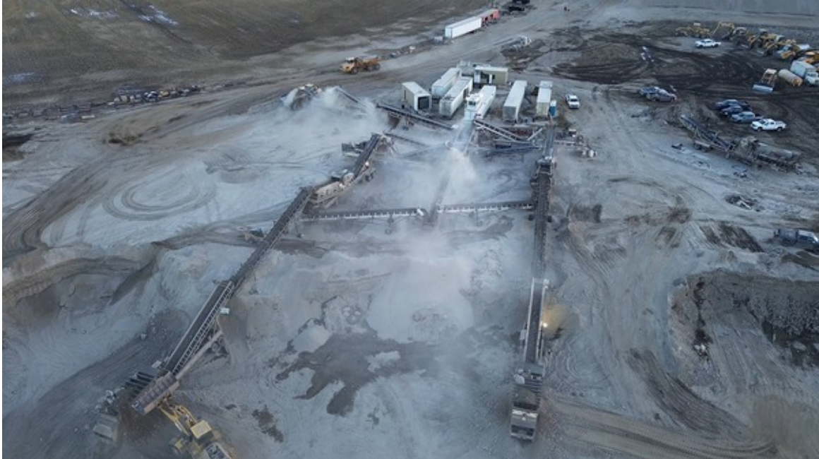
Gravel Crushing Commencing at Fincastle Pit Facing SW
