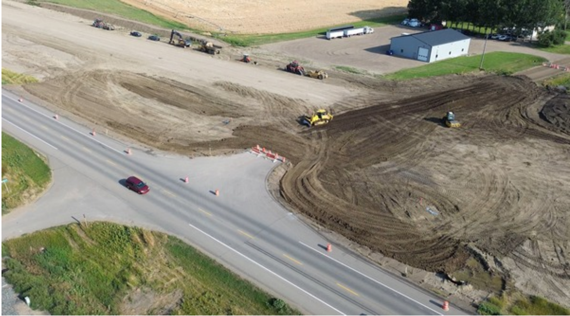
Intersection Widening and Subcut at RR 163 Facing South
