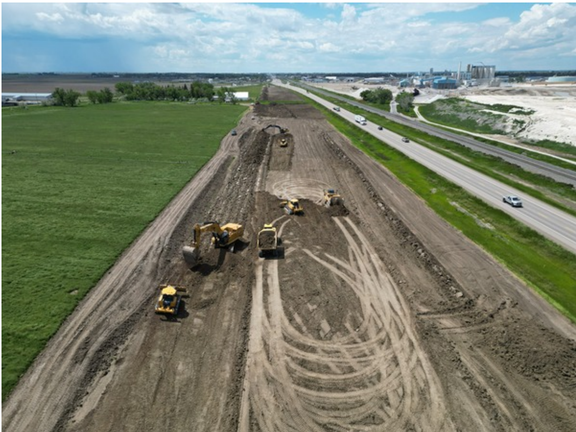
Ditch Cut and Subgrade Construction Between Taber and RR 163 Facing West
