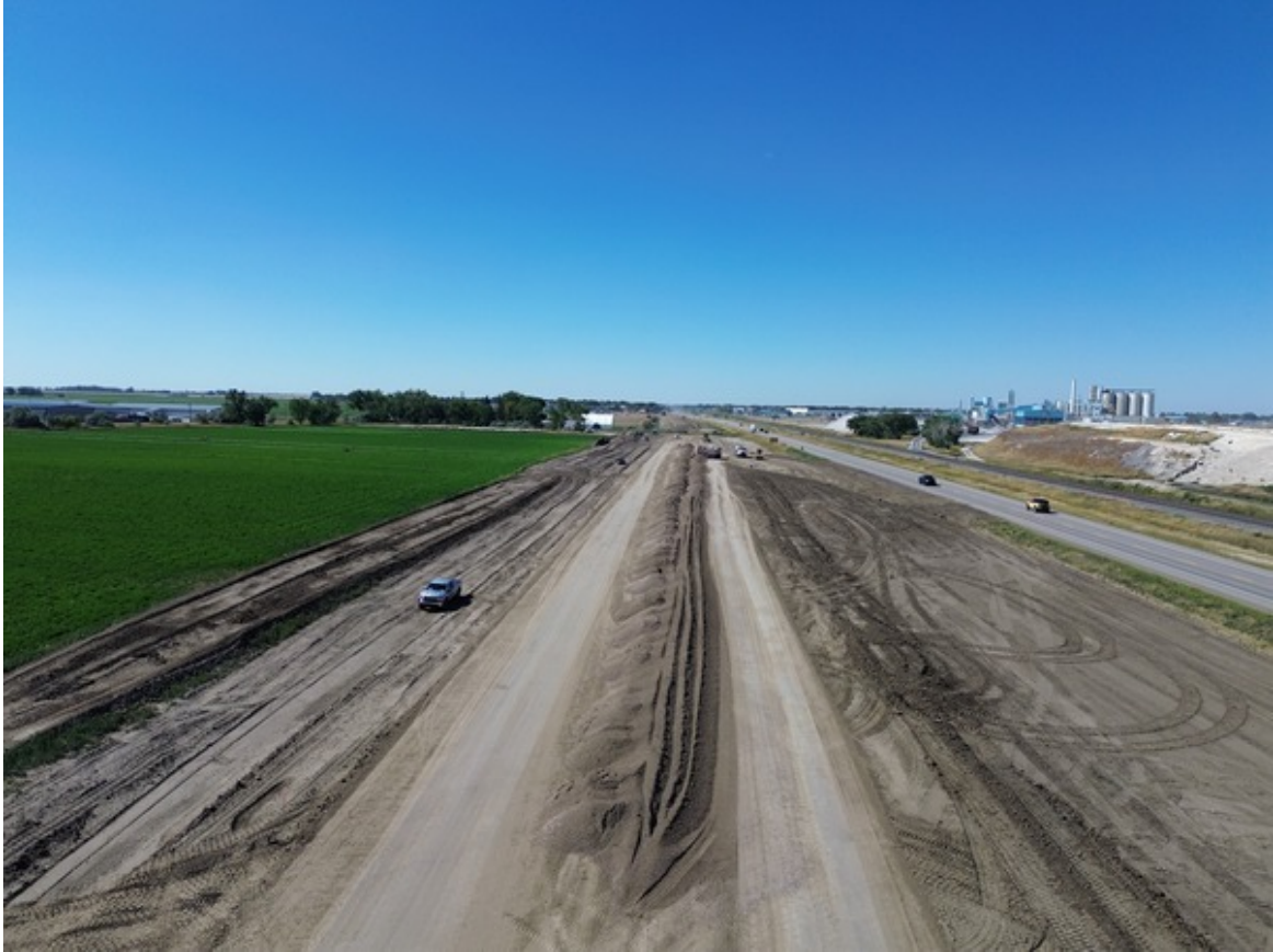
Gravel Placement Between Taber and RR 163 Facing West
