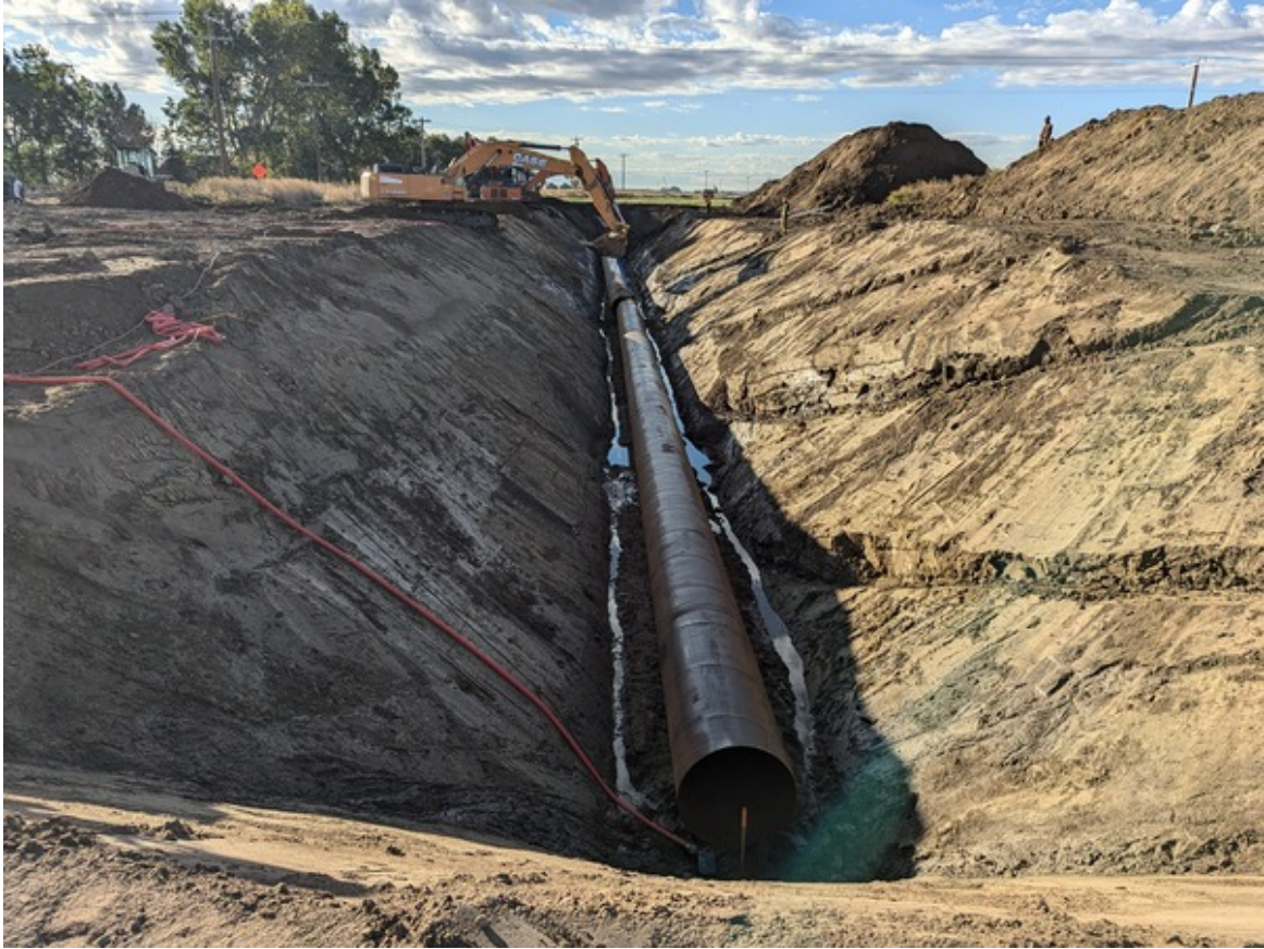
Lateral 20 Future Pipeline Casing Between RR 154 and 155 Facing South
