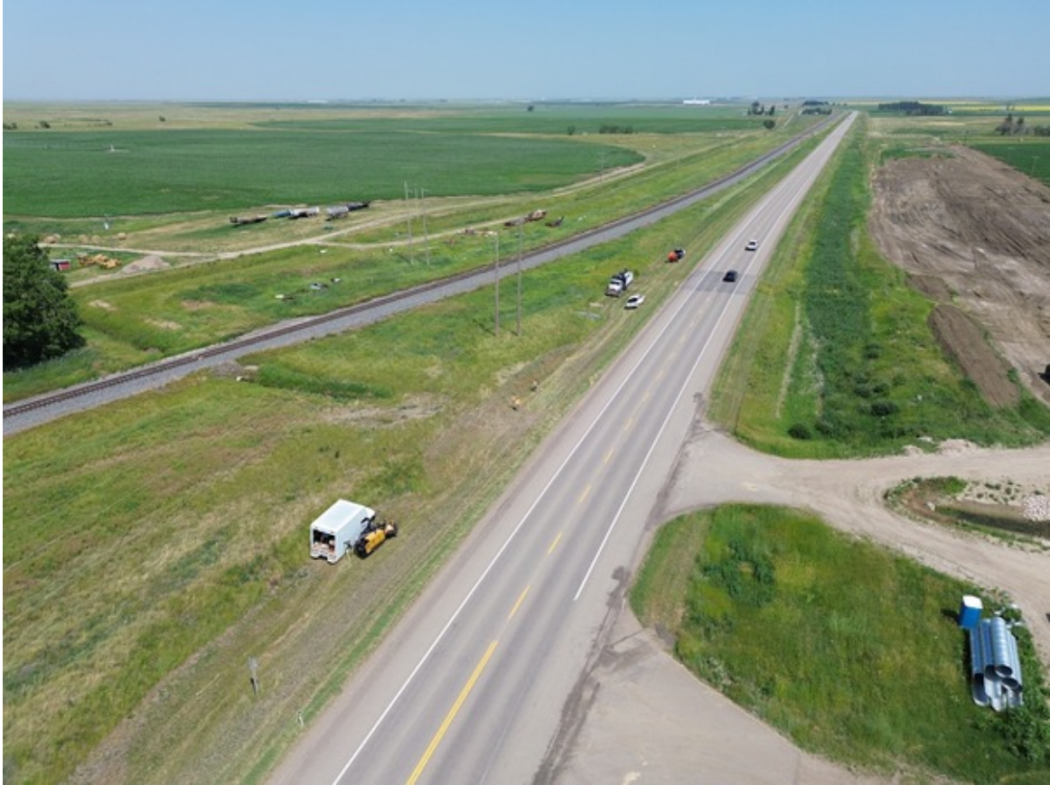
Fiber Optic Relocation East of Purple Springs Facing East
