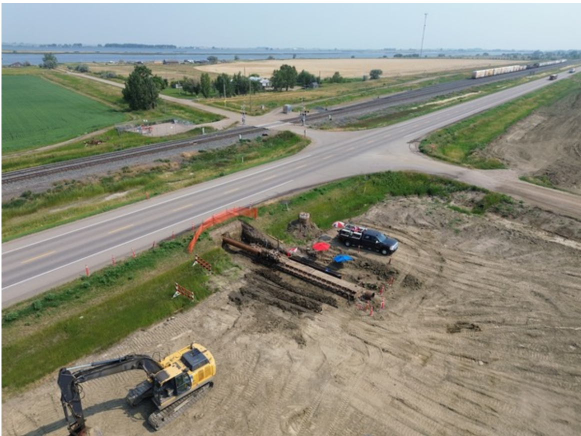
Culvert Bore Beneath Existing Highway at RR 163 Facing NE
