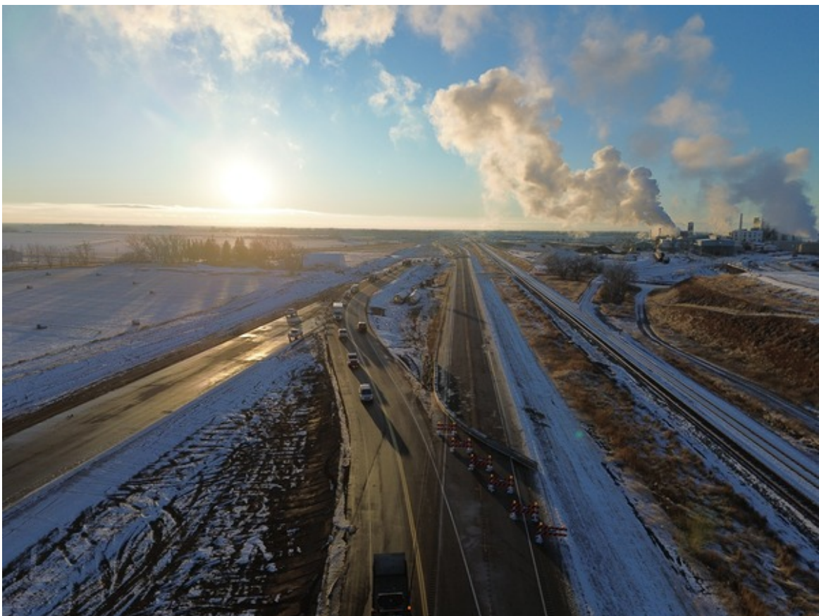
Detour 1 Implementation at Structure 1-2 Between Taber and RR 163 Facing West
