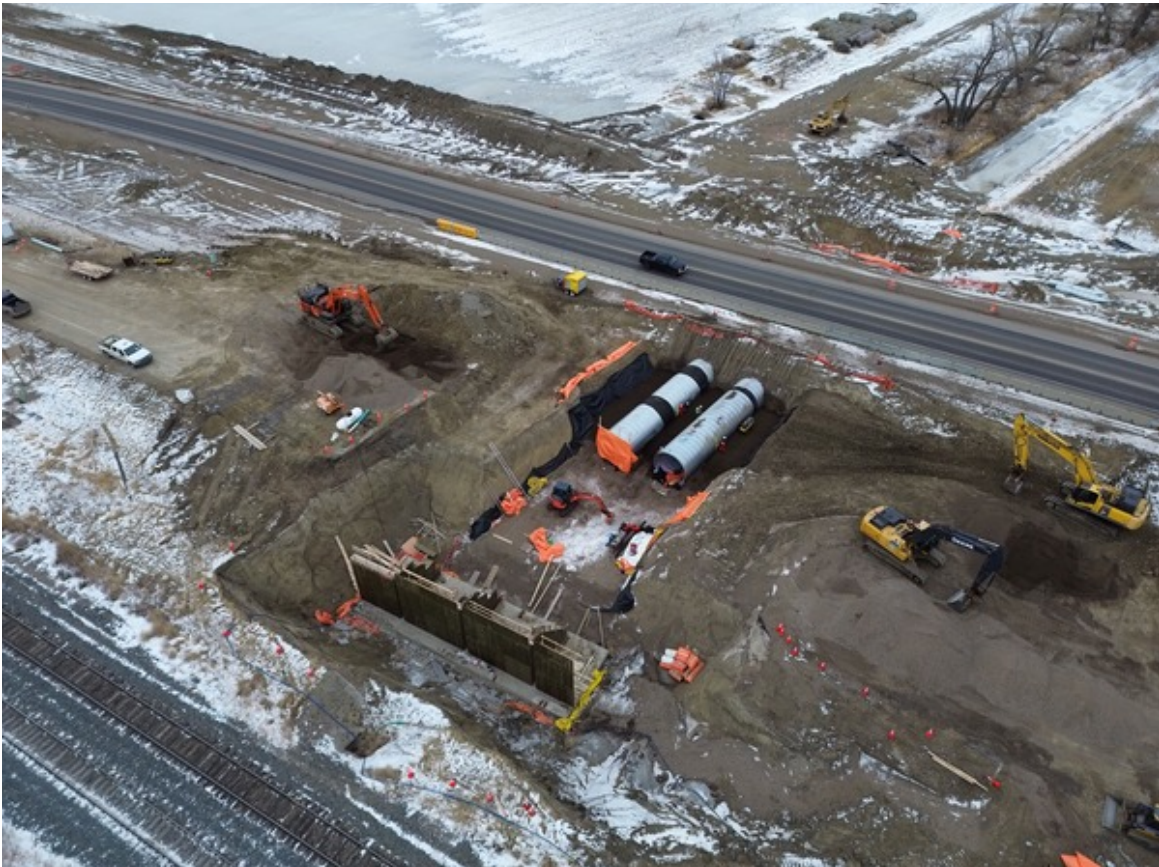
Backfilling and Placing Form Work on Structure 1-2 Between Taber and RR 163
