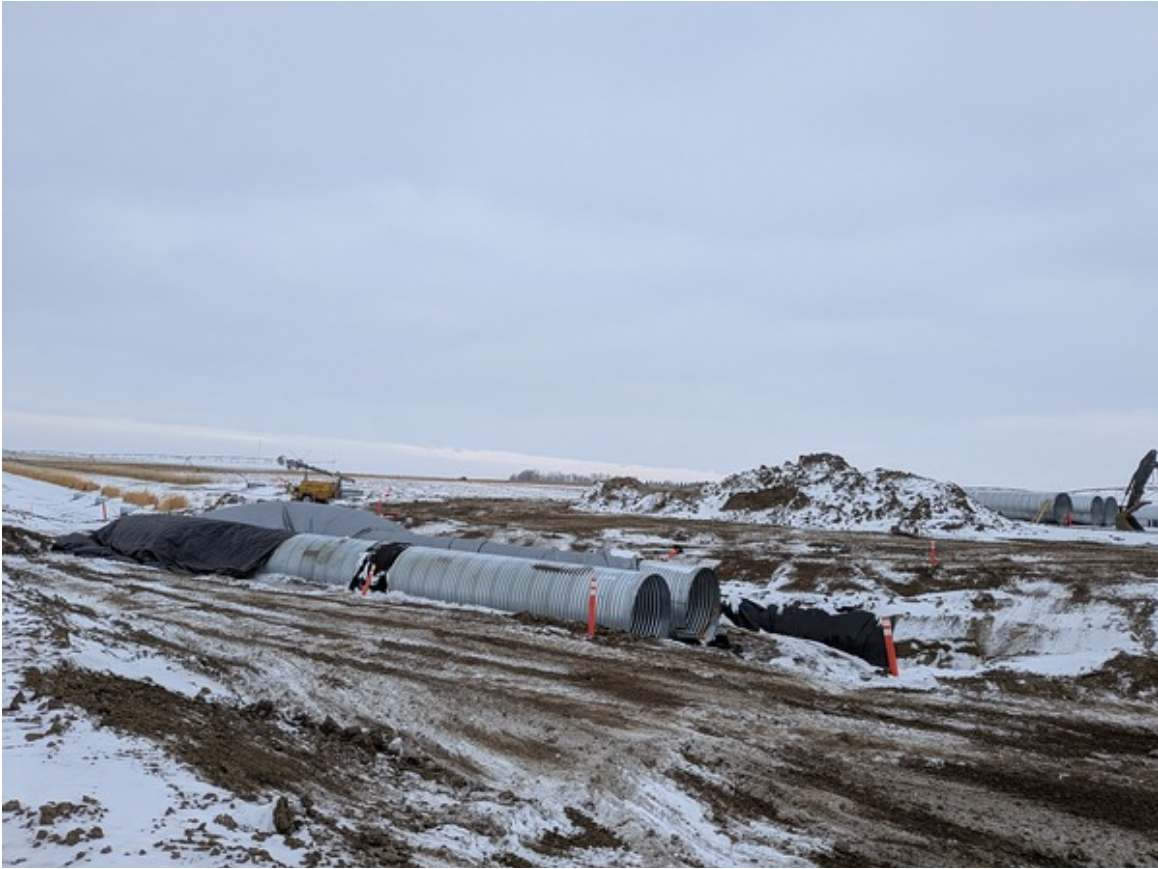
Heating and Hoarding of Structure 9-10 South of Grassy Lake
