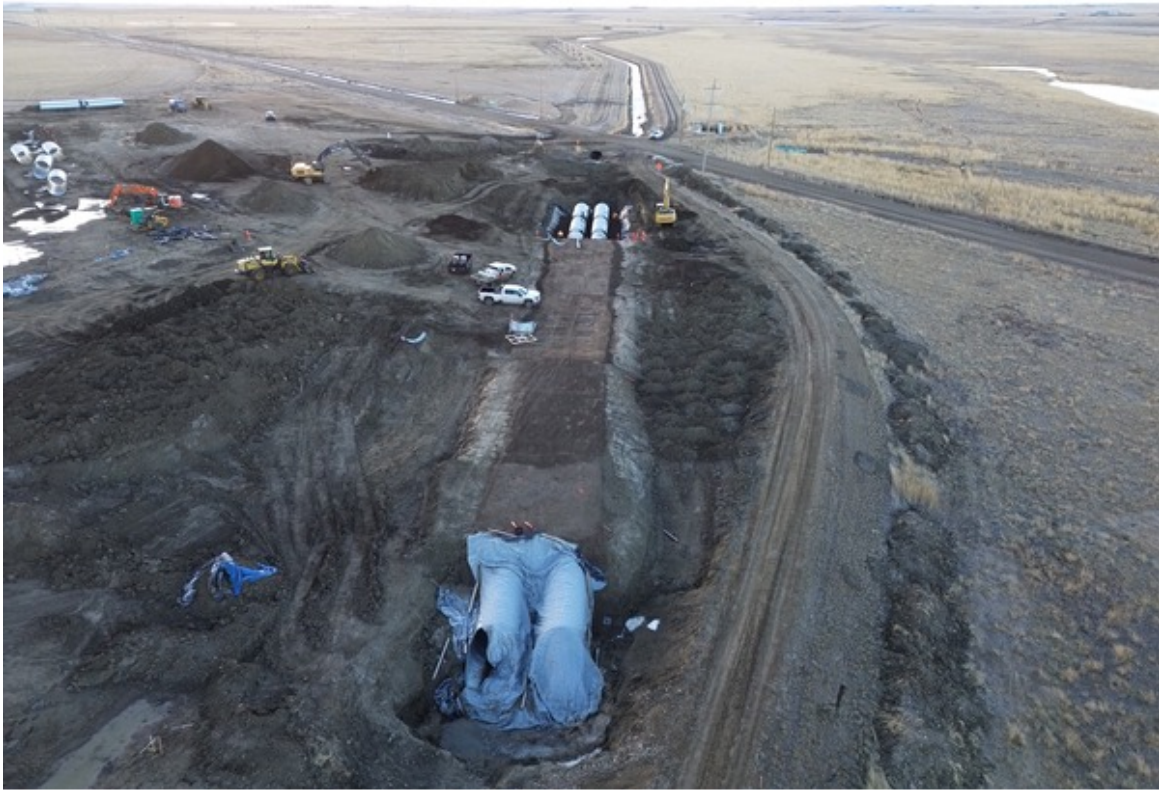
Backfilling and Setting in Pipe at Structure 9-10 South of Grassy Lake
