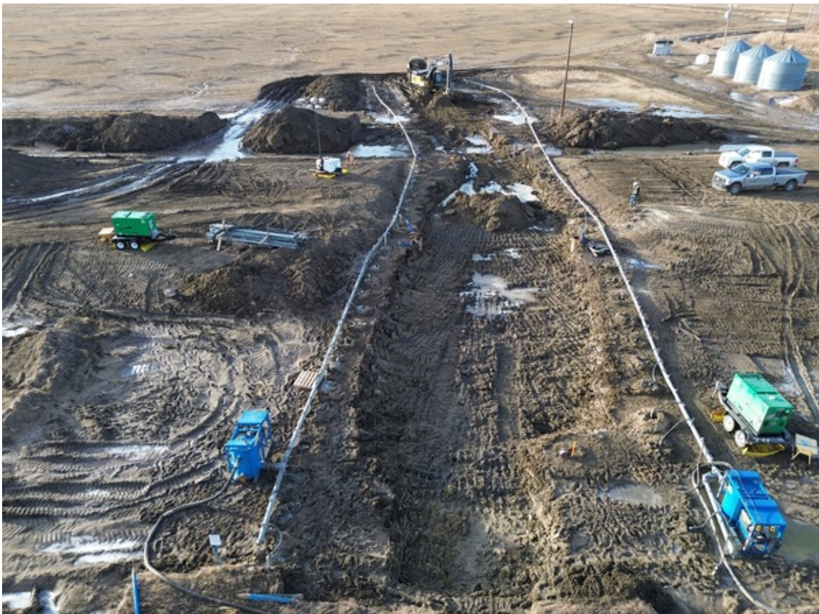
Dewatering at East Horsefly Main Pipeline Between RR 150 and 145
