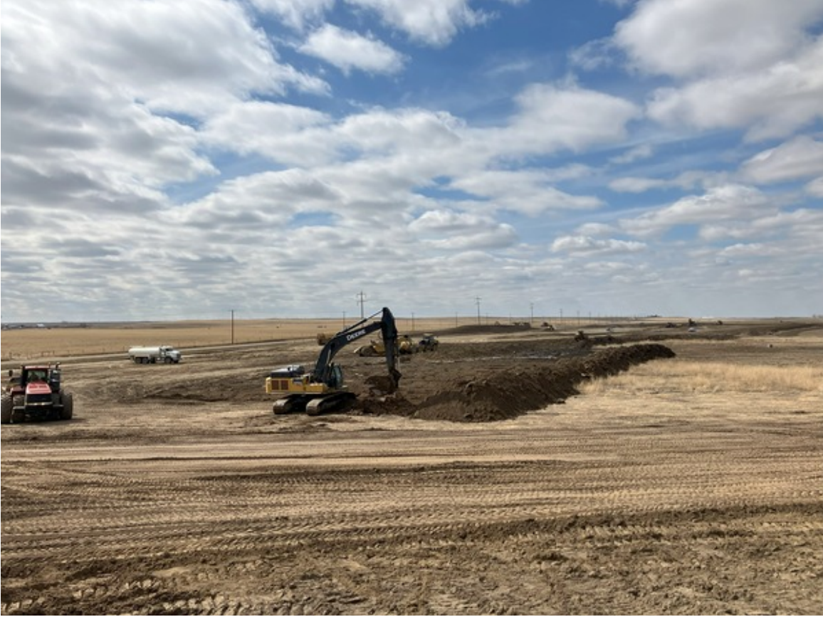
Earthworks Beginning in By-pass South of Grassy Lake
