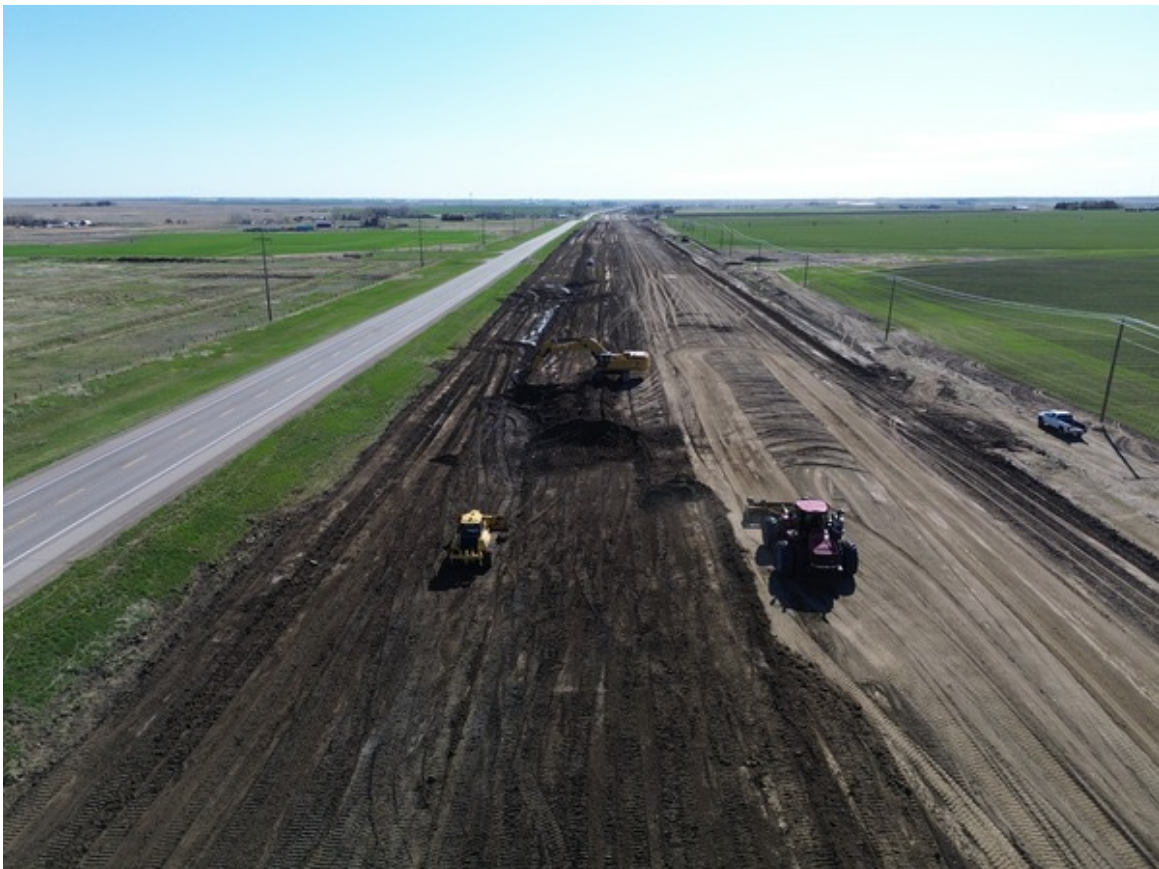
Completing Deep Median Ditch Cut Between RR 151 and 150
