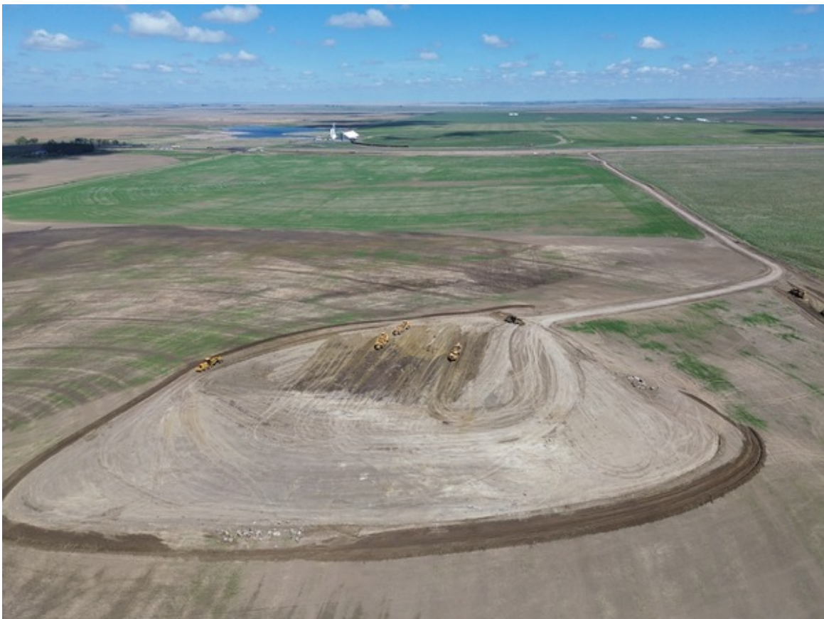
Grade Crews Building Subgrade from Borrow Pit Between RR 143 to 141
