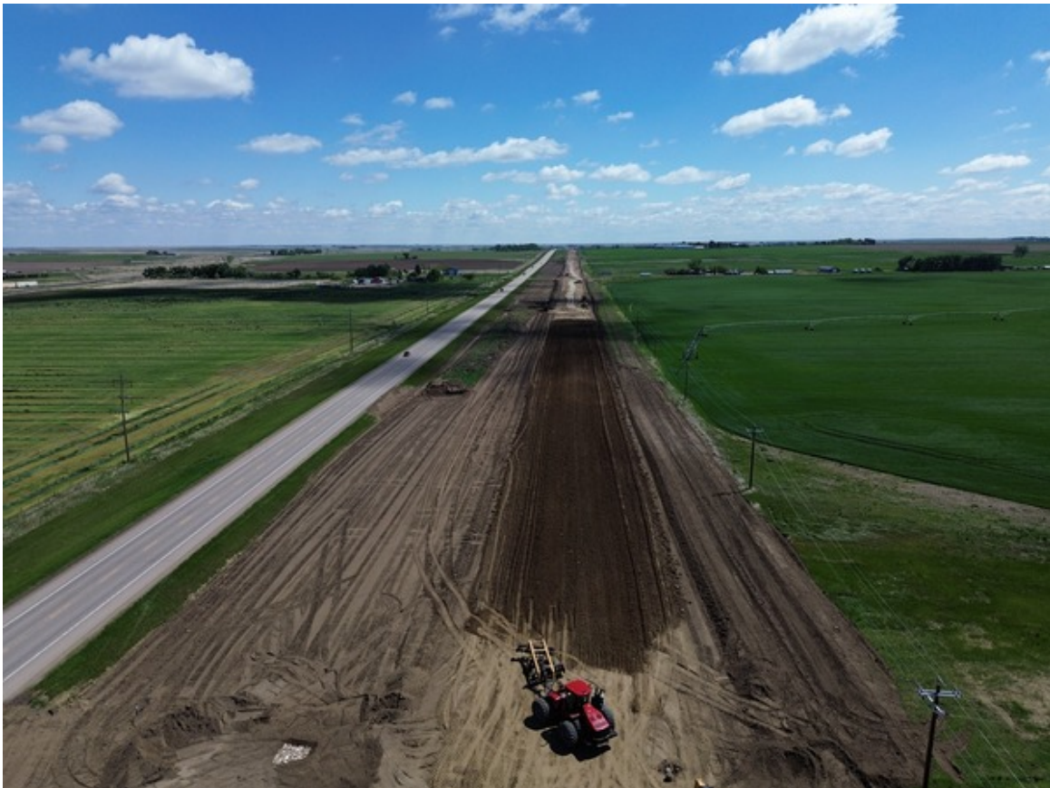
Final Subgrade Prep Between RR 153 to 152
