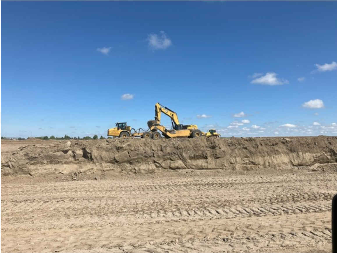
Crews Completing Deep Subcut in Bypass South of Grassy Lake
