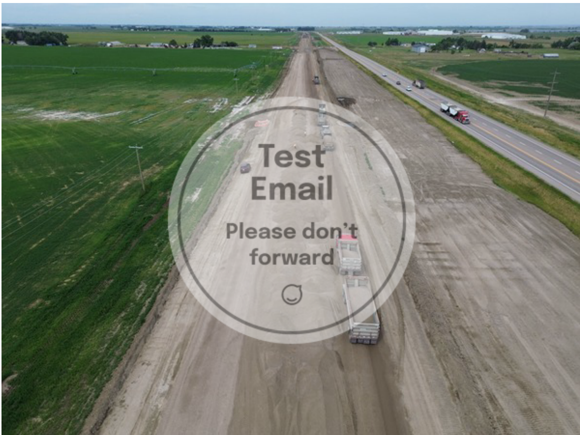
Gravel Crews Placing 2nd lift of GBC Between RR 152 and 151
