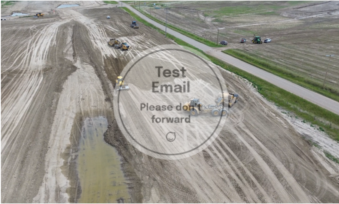
Grading Crews Placing Material in Deep Fill Section South of Grassy Lake
