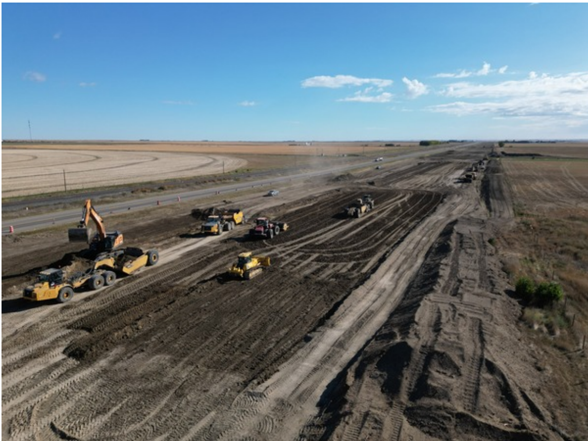
Grading Crews Installing Twin Centerline Culverts on Existing Highway 3 Curve Realignment Between RR 144 and 143 Looking West
