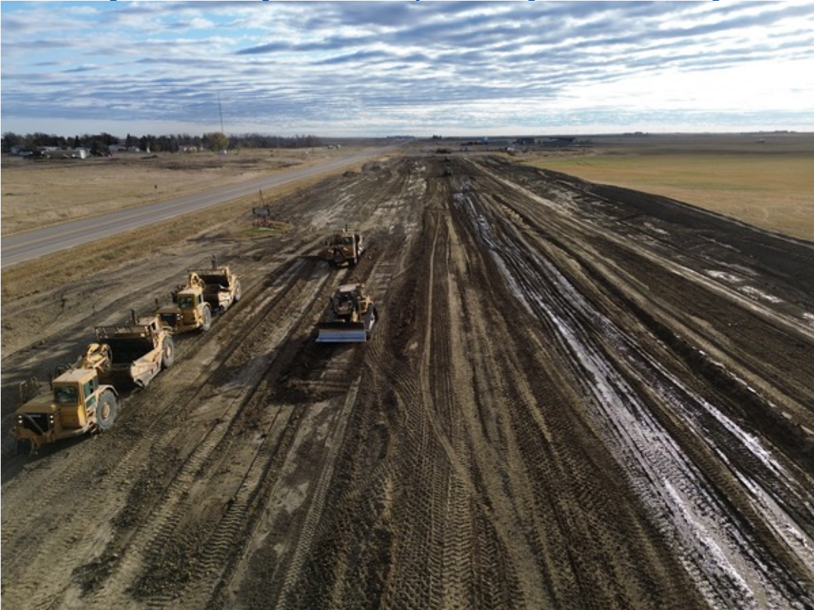
Grading Crews Working on East Grassy Detour Leg at RR 132 Looking East
