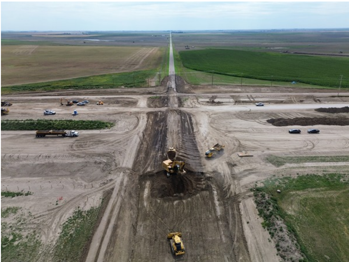
Crews Installing Twin 3.6m Culverts with Concrete Headwall East of Taber on Temporary Detour
